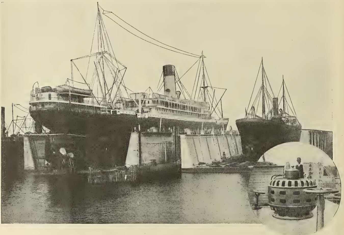
Fig. 6.—24,000-Ton Dock of the Robins Dry Dock & Repair Company. Insert Shows One of the Twelve 100-Horsepower Westinghouse Pump Motors
